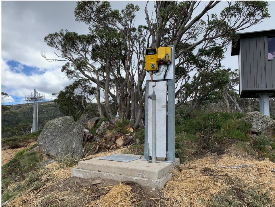
Image 5 - Example of prefabricated concrete pit, with hydrant and power outlet.
