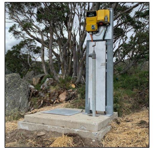
Typical Hydrant Arrangement
